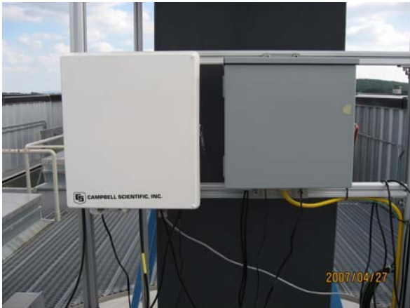
Figure 6 Datalogger box and power box installed on roof tower.
