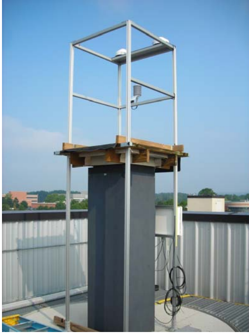
Figure 1 Roof tower with pyrgeometers and relative humidity sensor installed.
