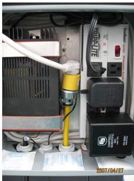
Figure 8 Interior of power box.
