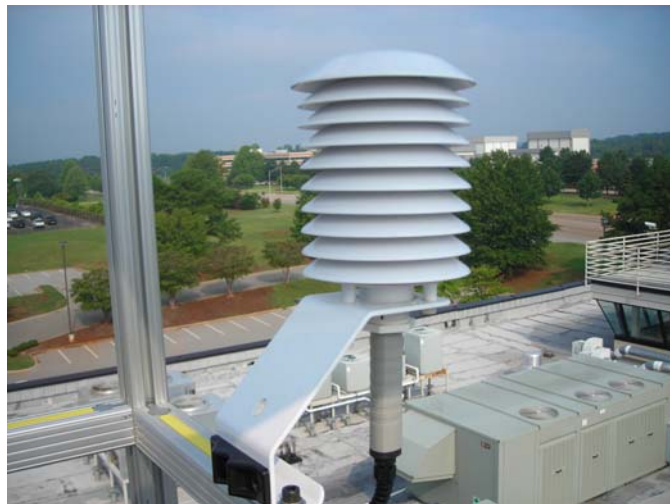
Figure 5 Relative humidity sensor installed on roof tower.
